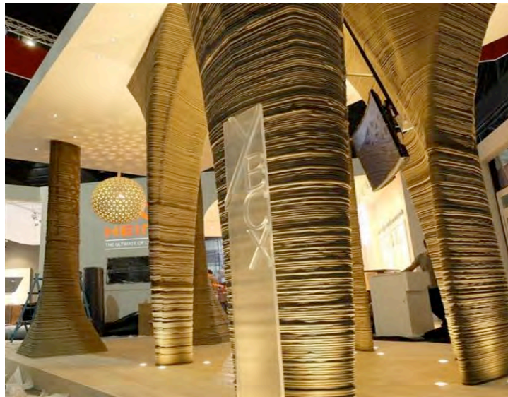
Figure 3. A 3D printed pavilion with very interesting spaces and volumes by SCG Thai cement maker.
