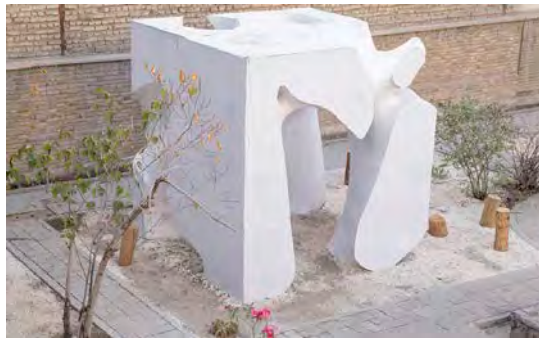
Figure 6. Craft Pavilion made with thin layer of fiber composite
