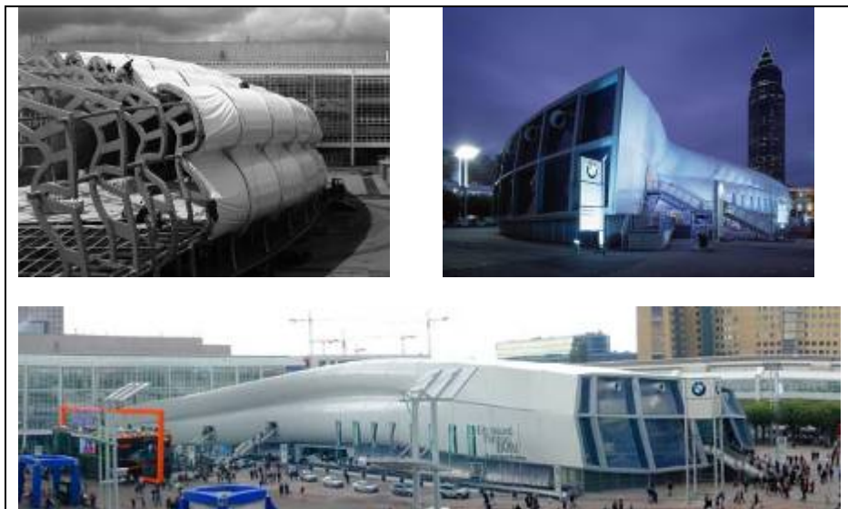
Figure 14 Because of its "moving" shape, the facade is covered by a one-layered printed Hostafalon ETFE membrane. The smart membrane details, such as supports of the clamping plate's door edgings, ETFE-fixation systems made this building a great success for the client Source: http://www.gregull-spang_de_content-Referenzen-Bilder-Messehallen-BMW.htm
