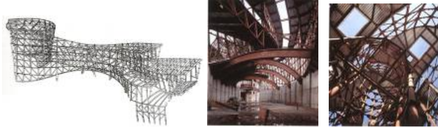
Figure 9 Guggenheim Museum in Bilbao, the 3D model and the assembly of its components Source: LeCuyer, Annette , "Building Bilbao" in Architectural Review, 1997
