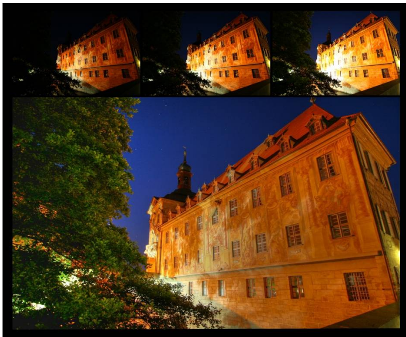
Figure 5. a.) to c.) Exposure set Historical Bridge City Hall, HDR-generation d.) Result with full contrast range.
