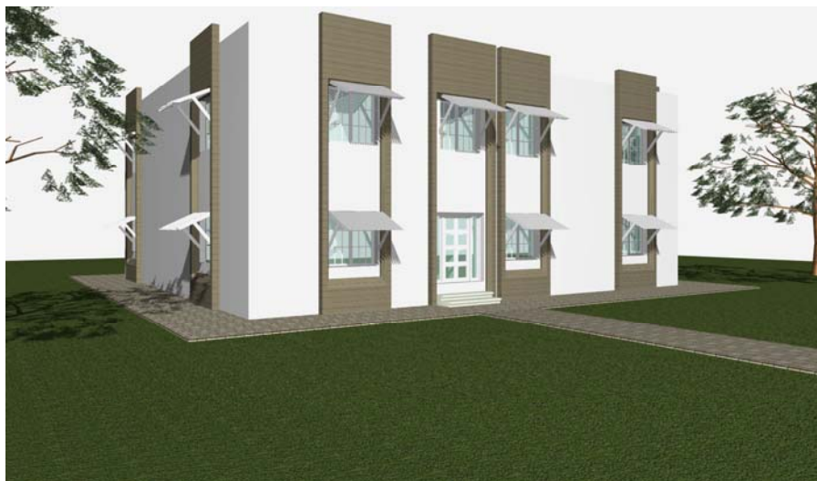
Figure 8. Simulation of Shading Devices as add-ons to the façade, overall perspective; Moza Alsuwaidi, Spring 2007
