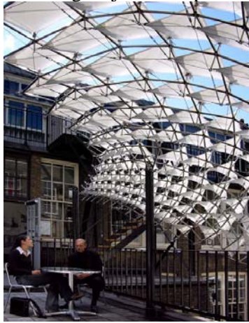
Figure 11. The Component Membrane Canopy constructed on a London roof terrace
