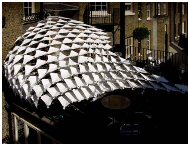
Figure 12. The Component Membrane Canopy structure
