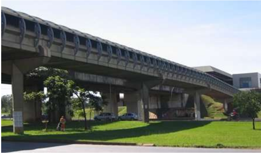
Figure 3. Pedestrian overpass – Metro of Brasília, structural design of Márcio Buzar (Source: http://www.cpcestruturas.com.br/ ).
