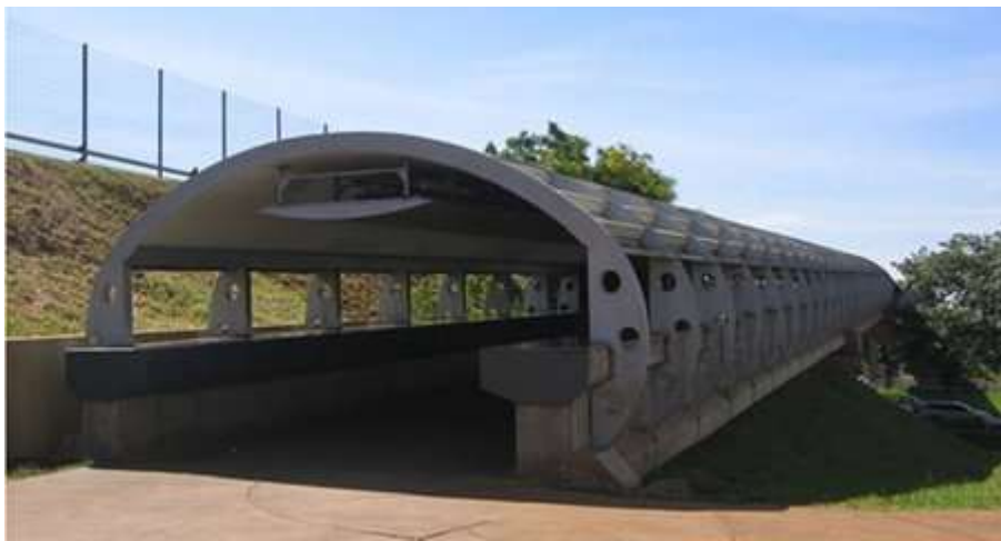
Figure 2. Pedestrian overpass – Metro of Brasília, structural design of Márcio Buzar (Source: http://www.cpestruturas.com.br/ ).
